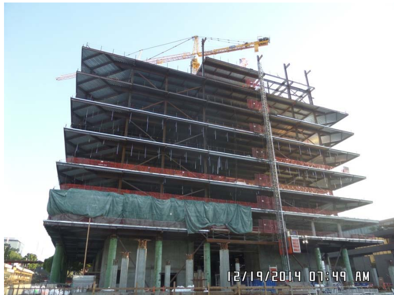
View of South Elevation
