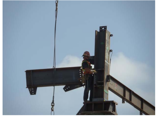
Temporary Column Connections
