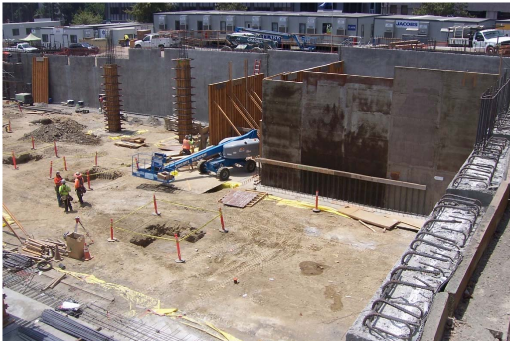
Generator Room Wall Forms
