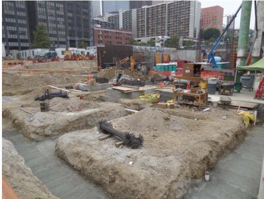
Transformer Yard Foundations
