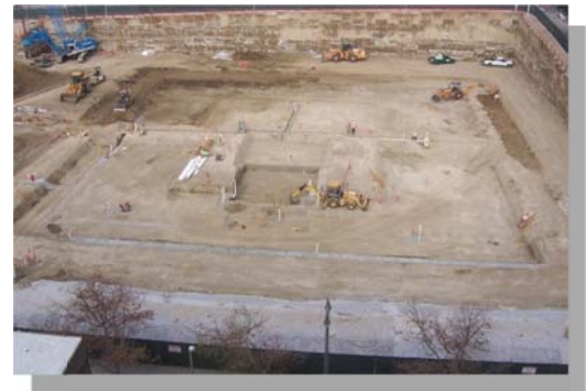
General Site Overview
