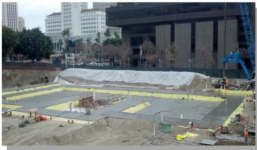
Start of Mud Slab Installation
