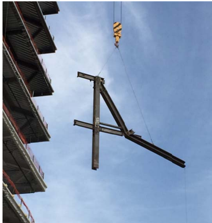
Roof Truss Pre-Assembly
