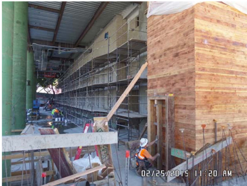
Board Form Installation
