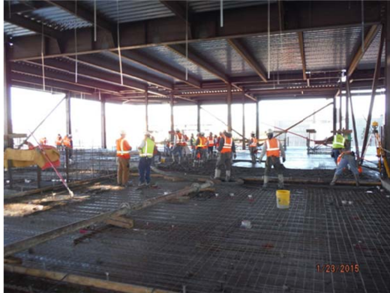
Placing Level 7 (West) Slab
