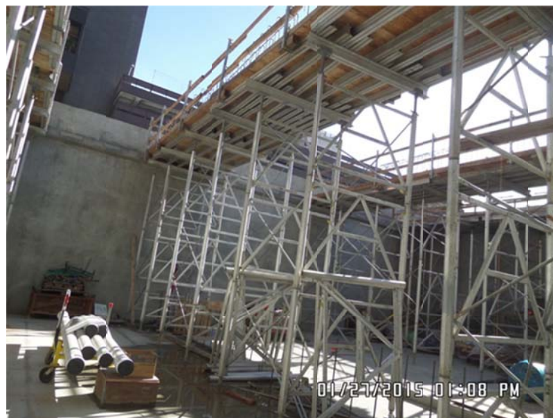
Shoring for Transformer Yard Structural Beams
