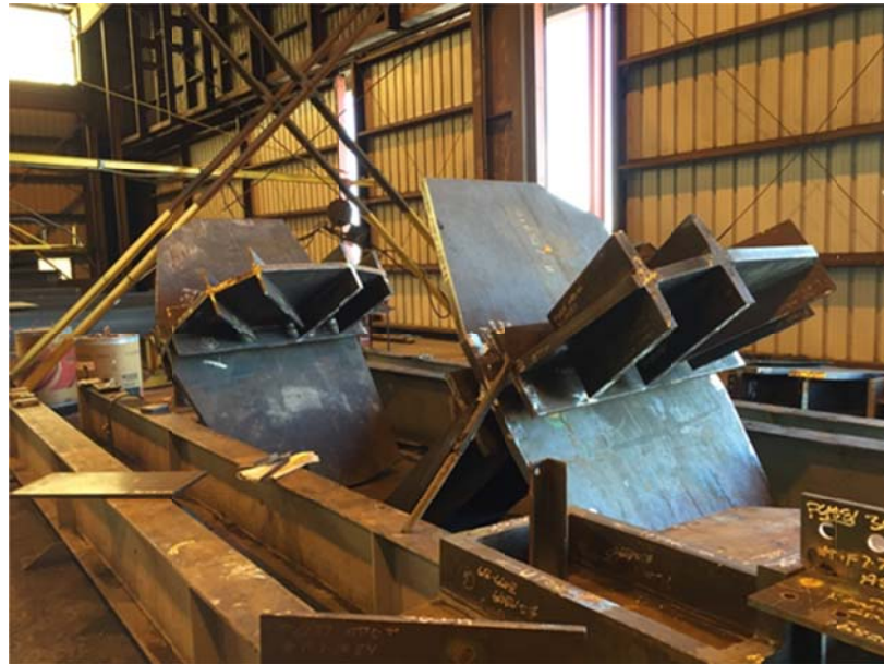
Roof Truss Fabrication
