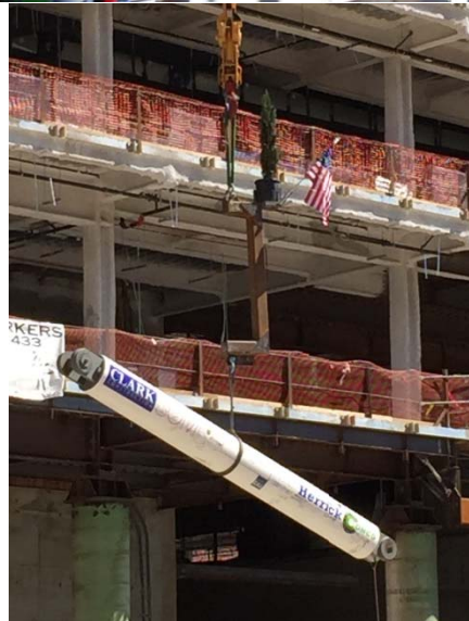
Topping-Out of the Structure
