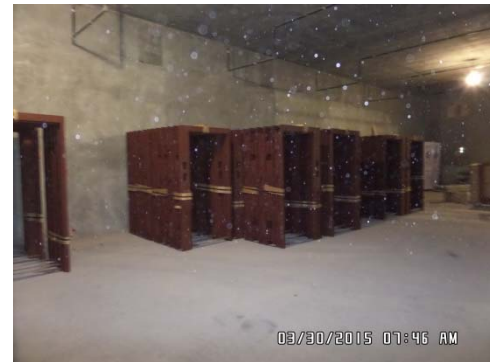
Detention Door Frame Delivery
