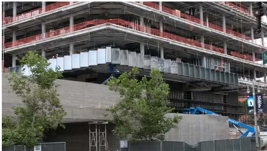
Curtain Wall Installation at Level 2
