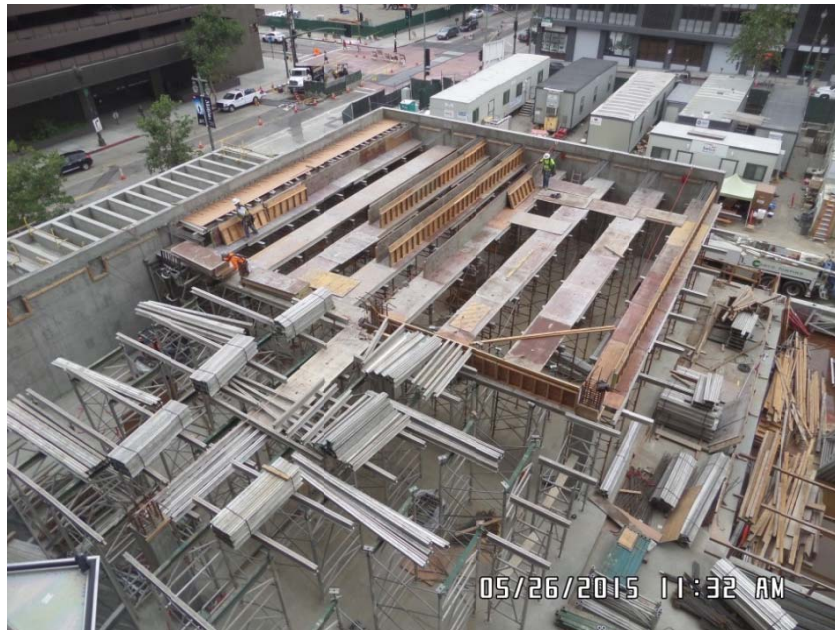
Jury Assembly Roof Formwork
