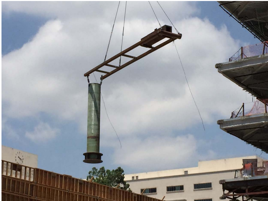
Removal of Temporary Column
