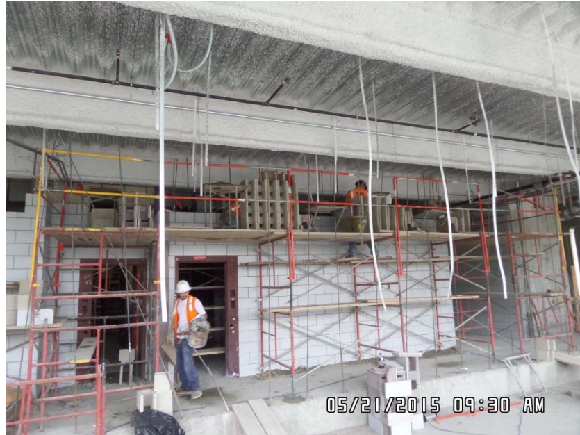
Glazed Masonry Installation – L3
